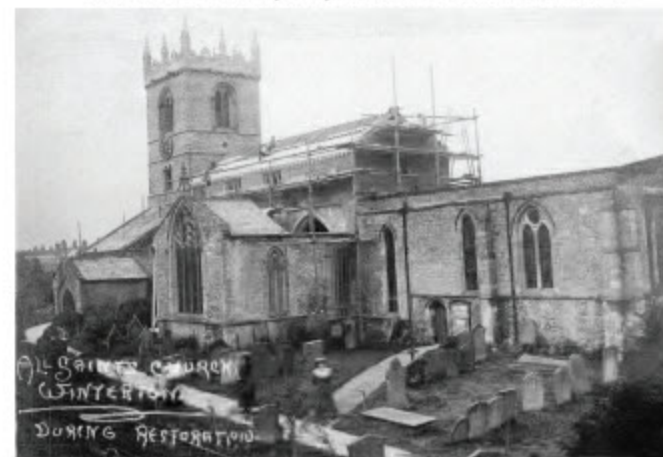
The Church during the 1904 restoration
